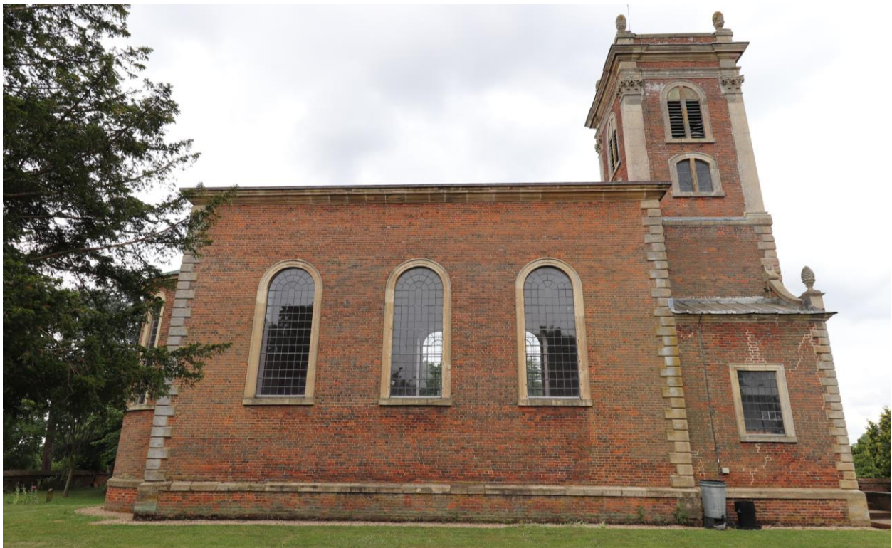
Above: North elevation of the church
