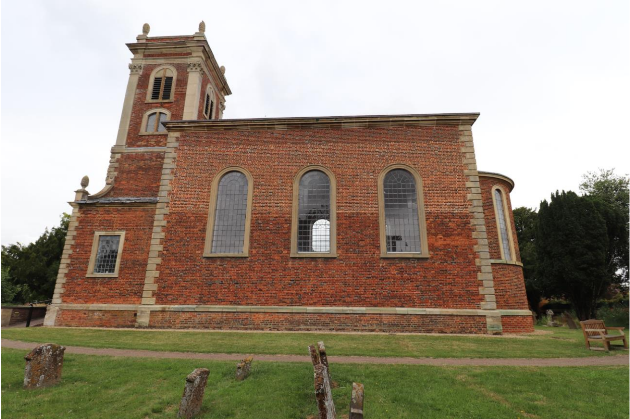
Above: South elevation of the church. Note the jarring effect at high level on the nave wall, the result of a different pointing style
