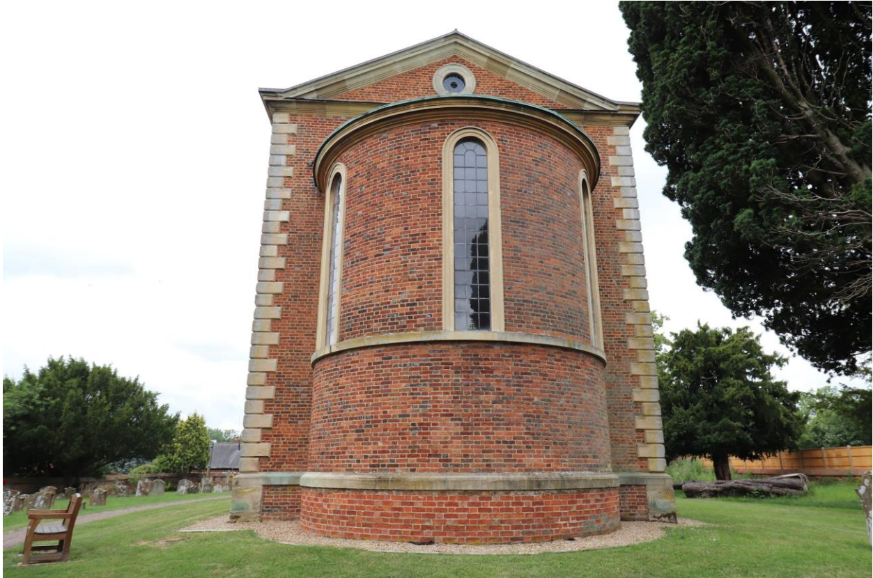
Above: East elevation of the church with apse of c. 1862. Note the different brick below plinth level
